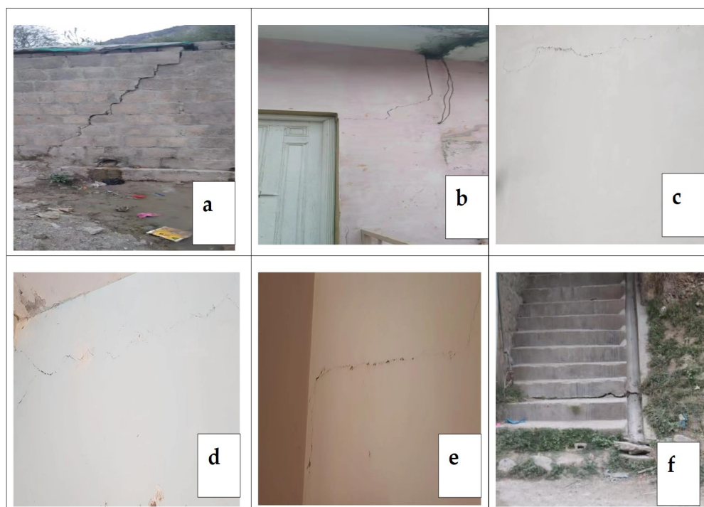
Figure 14. Cracks in the walls and stairs within the study area (a–f).
