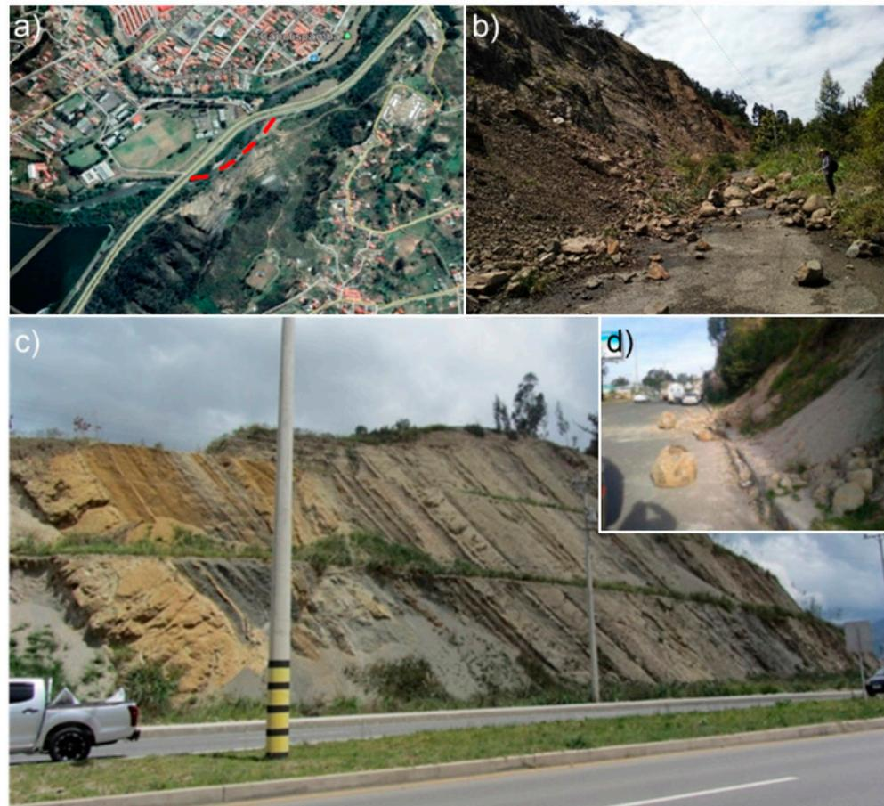
**Figure 2.** The functionality of the Pan-American Highway is often interrupted by rockfalls. (a) Deviation of the original road axis (red dotted line) caused by rockfall events; (b) landslide deposits have almost completely invaded the highway; (c) over-dip cataclinal slope: the stratification is slope-oriented; (d) boulders detached from the slopes block the lane.
