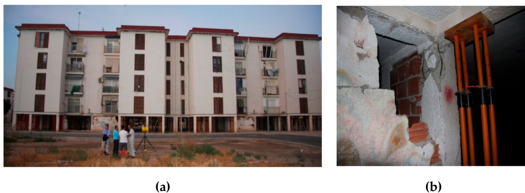
Figure 3. (a) Typical buildings in San Fernando neighbourhood; (b) Example of a damaged pillar.
