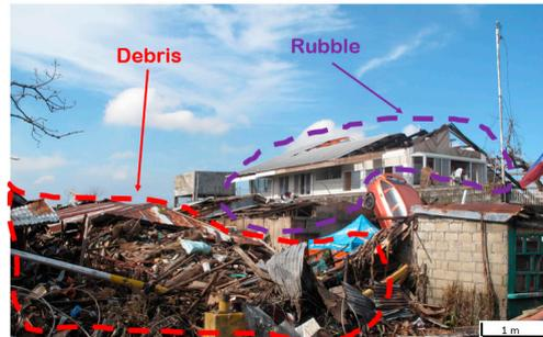
Figure 6. Damage classes: Examples of rubble and debris at the building level in Tacloban [32].
