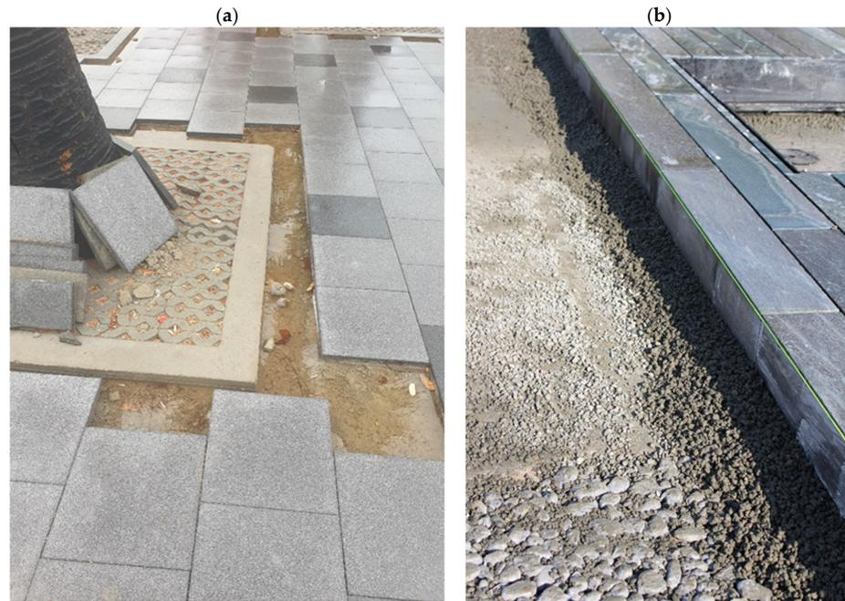
**Figure 5.** (a) Bound construction where pavement areas are placed directly on concrete slab and water will not drain, and (b) bound construction where pavement areas are placed on monograin concrete for drainage (photos by P. Petschek).
