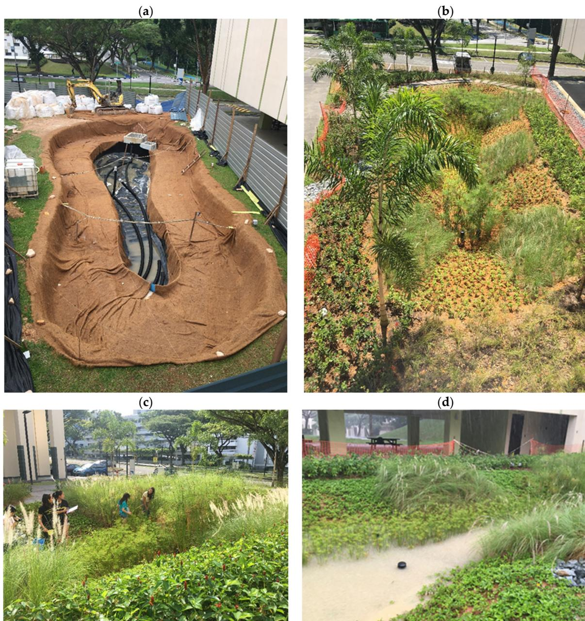
**Figure 8.** (a) Rain garden construction in Singapore showing geotextile and underdrain connecting to the discharge sump (left concrete sump) and overflow sump (right concrete sump), (b) vegetation coverage three weeks after planting, (c) vegetation coverage and infiltration measurements two months after planting, and (d) surface water storage storm event six weeks after planting (photos by K. Irvine).
