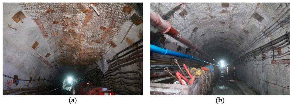
**Figure 21.** Roadway shape with or without fracturing and pressure relief: (a) unfractured section; (b) fracturing section.
