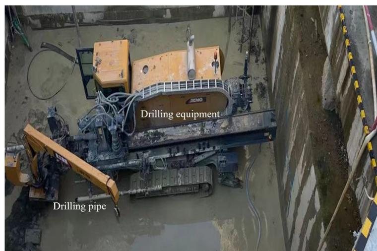
**Figure 8.** Horizontal-directional drilling applied for the multi-pilot heading pretreatment used in the pipe jacking engineering.
