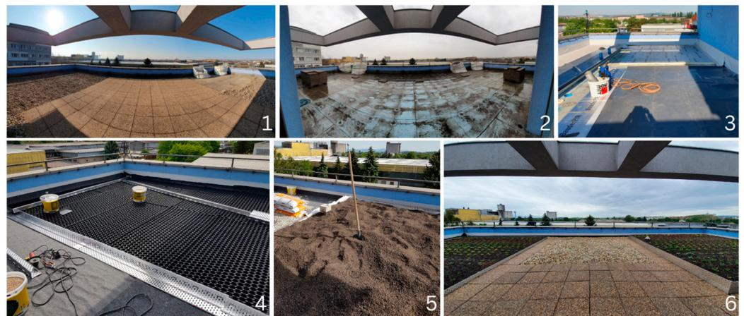
**Figure 3.** Photographs of the construction of the experimental green roof with biodiversity potential. 1—original state of the terrace; 2—removal of unwanted layers; 3—adding an additional thermal layer, a new waterproofing layer, and application of the measuring infrastructure; 4—installation of protection, drainage, and accumulation layers; 5—distribution of the substrate; 6—experimental roof after completion of construction works.
