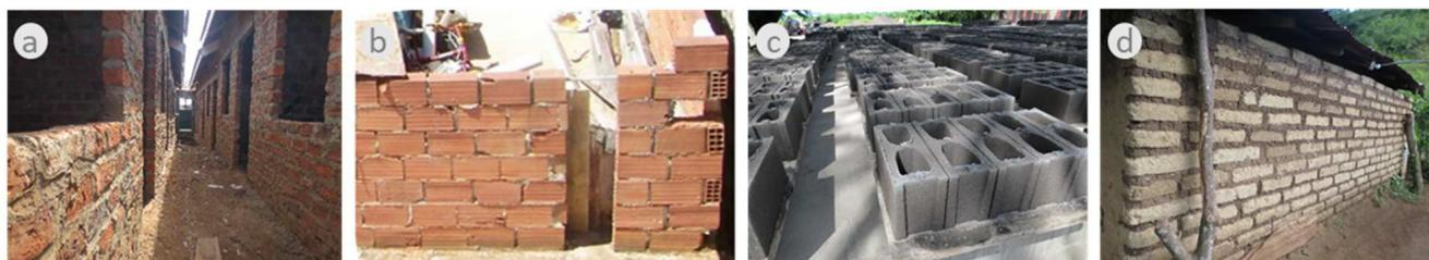
**Figure 1.** Mainstream building materials for walls used for low-cost housing: (a) fired brick wall in Uganda; (b) wall of hollow terracotta bricks in Brazil; (c) hollow concrete blocks for housing in Nicaragua; (d) wall of adobe blocks in El Salvador. Sources: Bredenoord.
