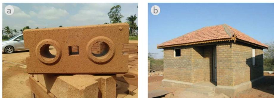
**Figure 7.** (a) Contemporary CSEB used in Gujarat; (b) wall with CSEB built for housing in Gujarat (2002). Sources: (a) Indiamart.com; (b) Catholic relief services.
