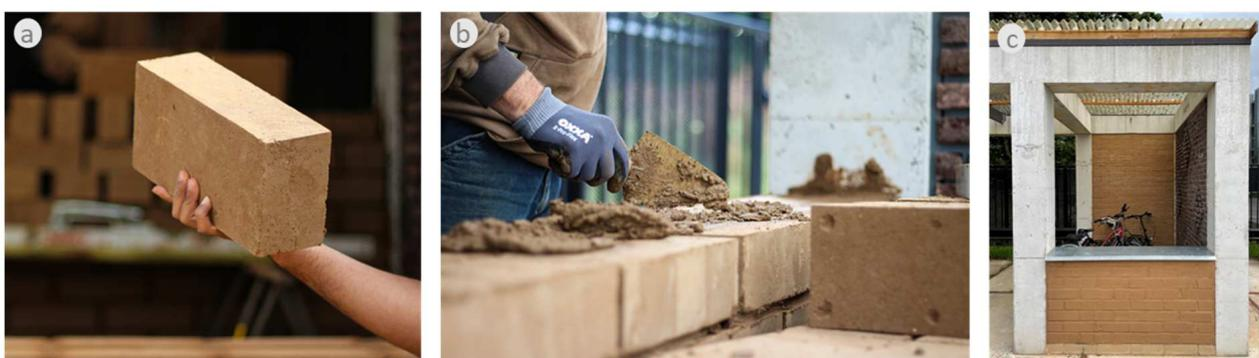
**Figure 13.** Cow-dung stabilised CEB wall constructed at TU Delft, Netherlands provide evidence of its water resistance characteristics in the rainy weather of Netherlands. (a) Cow-dung stabilised CEB block, (b) Cow-dung stabilised earthen mortar, (c) Cow-dung stabilised CEB wall. Source: Kulshreshtha.
