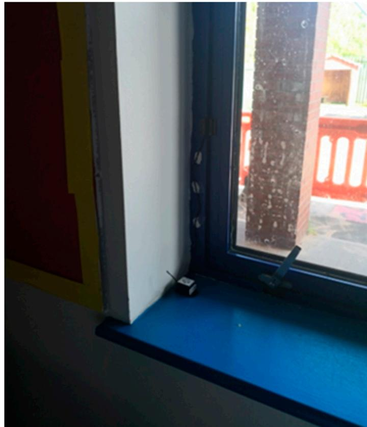
Figure 33. Window open/closed status installed sensor in School A.
