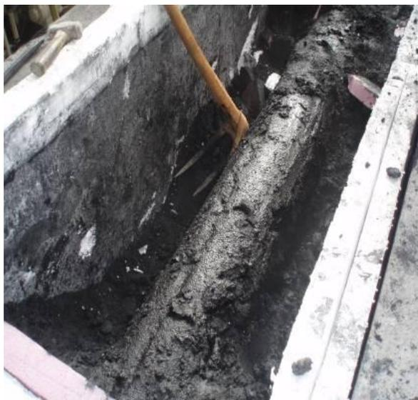
**Figure 5.** Freezing effect around freezing pipe.
