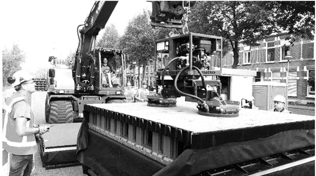
**Figure 2.** The currently available construction method of the prefabricated plastic panel for the cycle path (after [14]).
