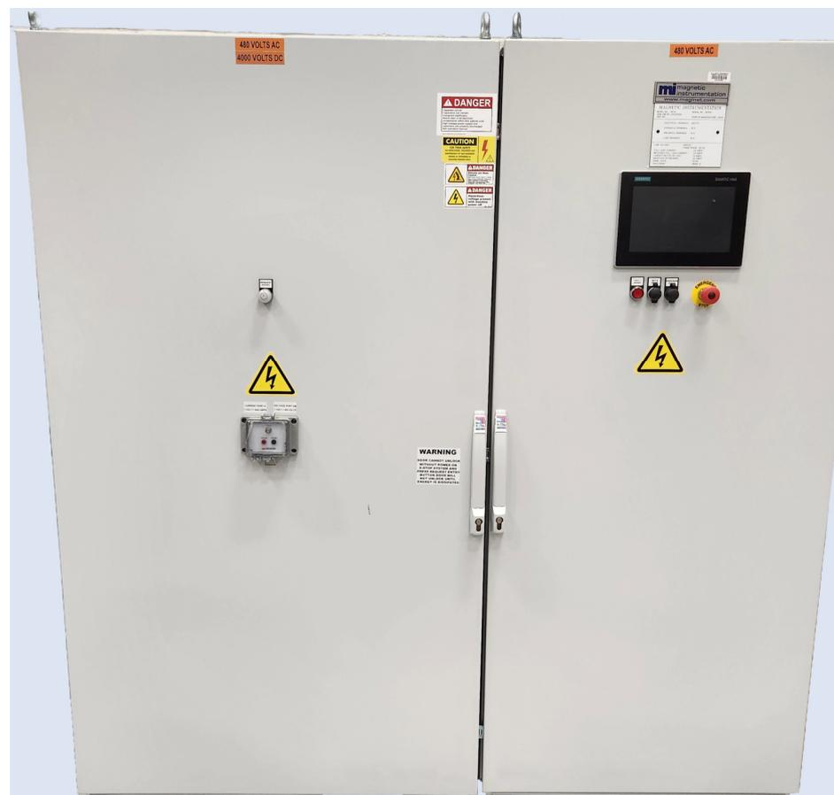
Figure 14. Image of typical pulsed magnetizer equipment.
