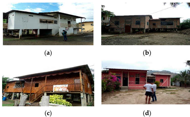
Figure 4. The construction materials used in the housing of the three spaces. (a) Reinforced concrete, (b) masonry, (c) wood, (d) others.
