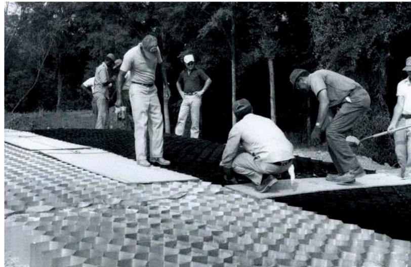
**Figure 1.** Early version of geocells used by US Waterways Experimentation Station at Vicksburg, MS, USA [1].
