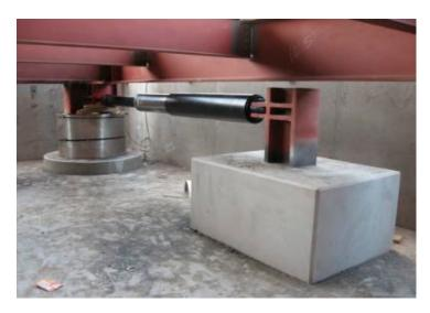
**Figure 6.** FVD's location in the isolated building [60].
