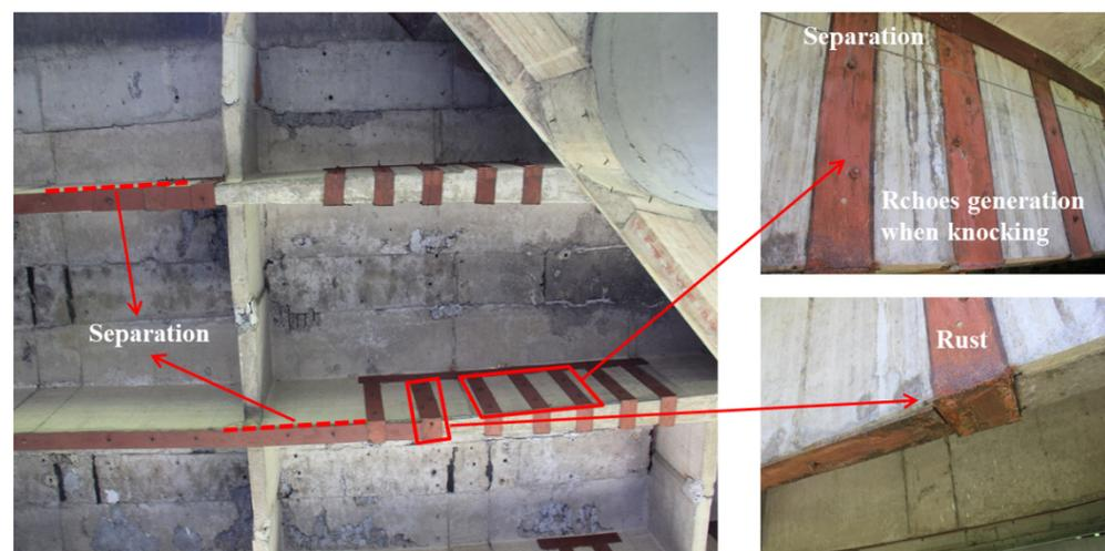
**Figure 3.** Damage to externally bonded steel plates.
