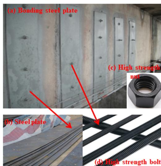
Figure 18. Bonded steel plate.
