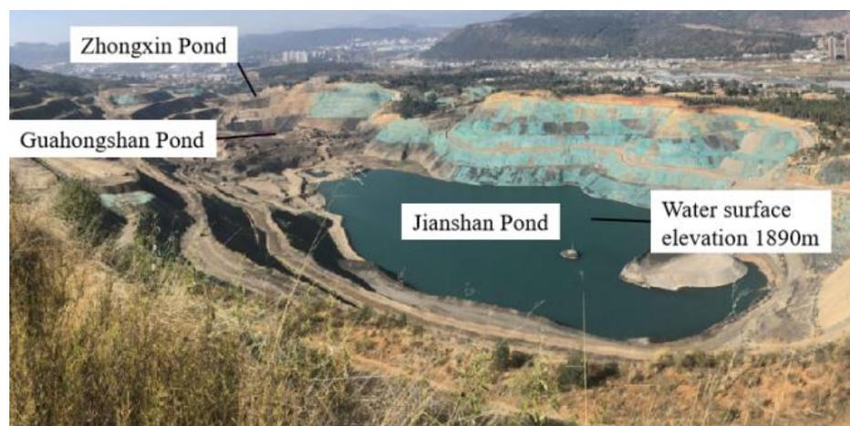
**Figure 1.** Water accumulation in the mine pit.
