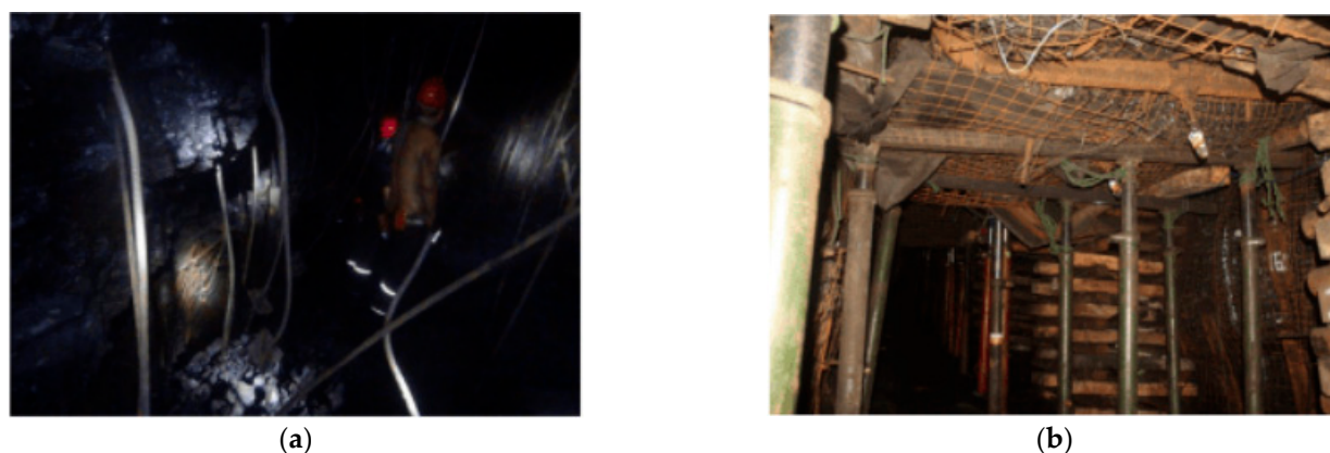
Figure 2. Scene damage of 20 October rock burst accident in Longyun Mine: (a) Anchor bolt bent and suspended; (b) Two sides convergence, roof subsidence.
