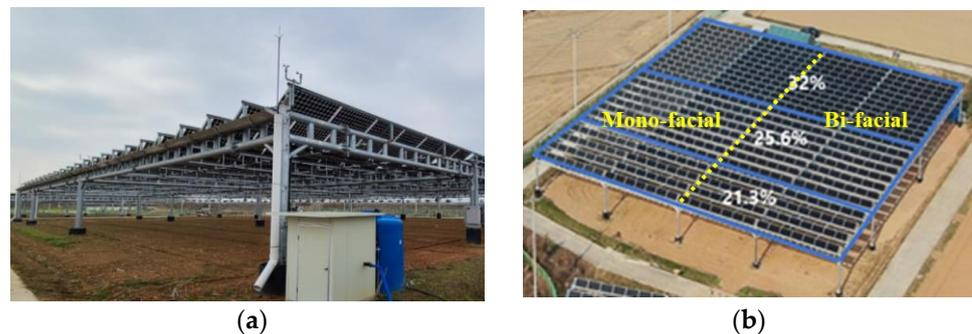
**Figure 1.** Tested agrophotovoltaic system: (a) overview; (b) APV with different module types (bi- and mono-facial) and shading ratios (21.3%, 25.6%, and 32%).
