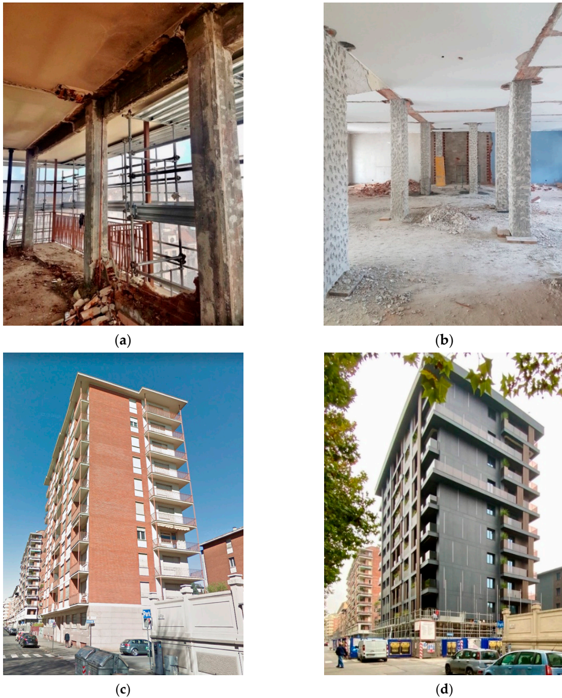
Figure 4. “The Black One”, images of the building site. (a) First phase of the building envelope’s substitution; (b) preliminary phase of the anti-seismic structural reinforcement; (c) the building before the retrofit intervention; (d) the building after the retrofit intervention (photo a, b by Lonero G.) [28].
