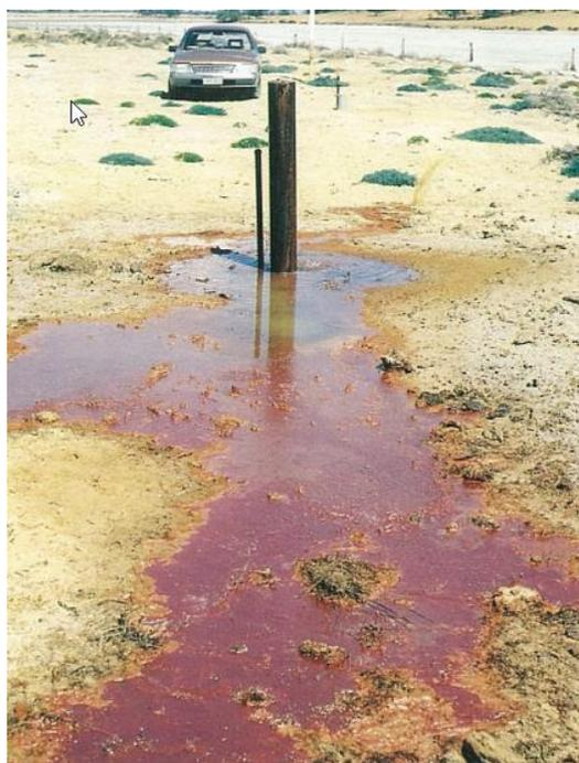
**Figure 20.** Iron-rich groundwater flowing from an artesian bore in NW Victoria. The previously white plastic standpipe is iron encrusted, attesting to the rapidity of iron clogging [8].
