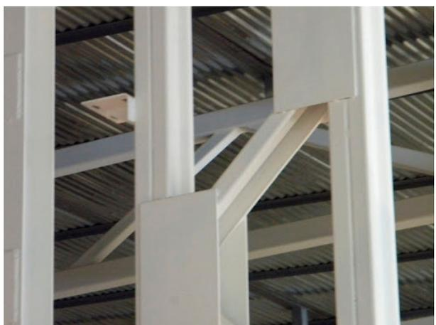
**Figure 2.** Vertical steel member fire protection.
