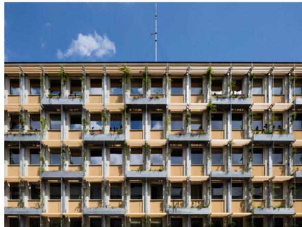
**Figure 1.** Frontal view of the renovated facade with trough-bound greening system [28]. © Rataplan Architektur ZT GmbH.
