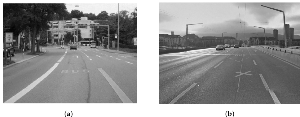
Figure 8. Within the city center, for example, approximately 20% of the lane-km are dedicated to public transport. Sources: [73] and Google Maps (a) discontinued bus lane upstream of an intersection and (b) special bus lane to bypass car queues.
