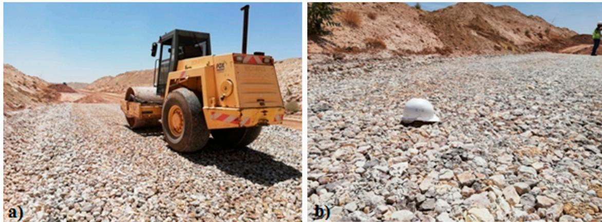
**Figure 6.** The appearance of the surface layer of the 25–100 mm aggregate size grading of SWR. (a) Poor granular arrangement observed during compaction; (b) dominant surface appearance at the end of the compaction, which reveals a high segregation phenomenon.
