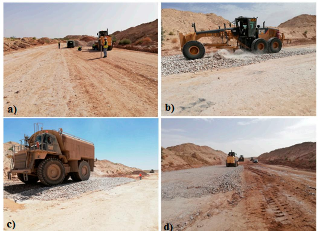
**Figure 5.** Various stages of the two full-scale field tests of the capping layers sections: (a) topographic layout and plate load test on existing embankment; (b) levelling with a grader; (c) watering the material up to WOPN; (d) compacting operation.
