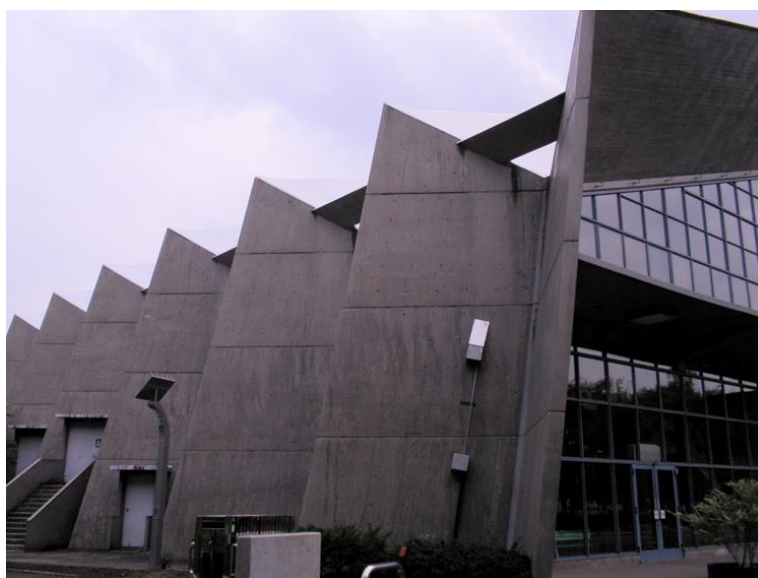
Figure 21. Folded V-shaped concrete sheets in the Performing Arts Center in Gunma, Japan. Source: authors.
