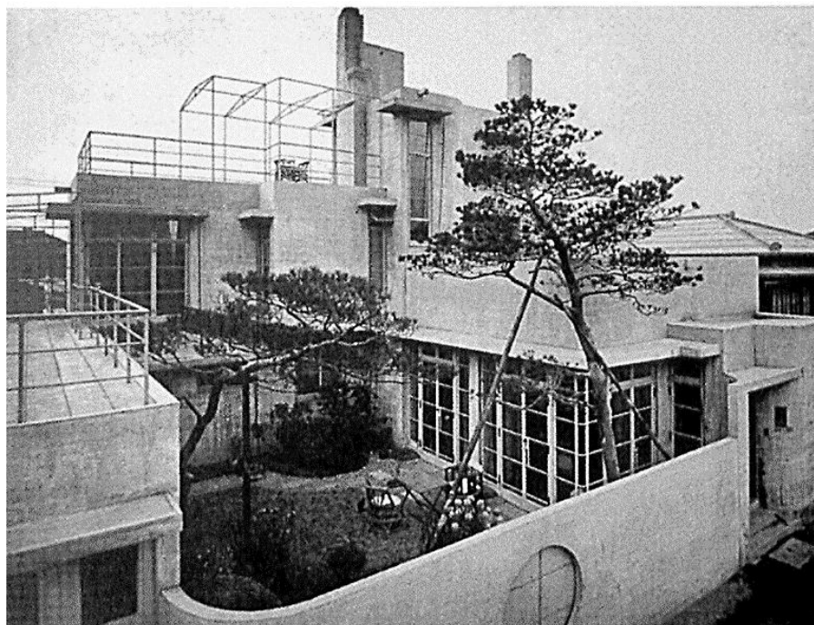
Figure 2. Raymond's Reinanzaka House in Tokyo, entirely realized in monolithic reinforced concrete (1923). Source: authors.
