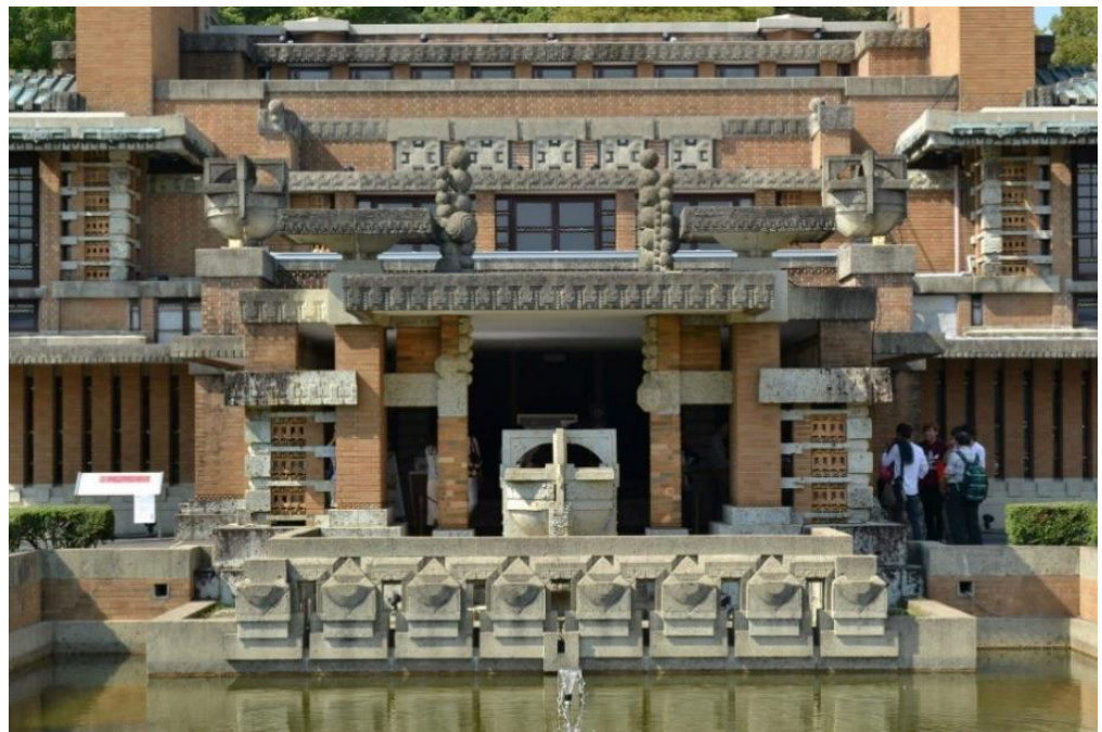
Figure 1. Imperial Hotel reconstruction at Inuyama (Gifu), showing masonry, excessive ornamentation and open disregard for local conditions and climate. 1—In grey: baubles and decorations in stone, resembling Mayan claddings. Stone is a very unusual material in façades in Japan, inadequate for resisting seismic forces and it was nowhere to be found near Tokyo. 2—In clay color: artistic brickwork which besides its rarity had already proven a failure on former buildings, especially when subject to earthquakes and other stresses. Source: authors.
