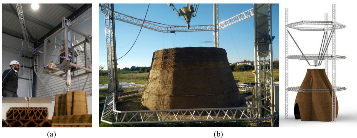
**Figure 9.** Cable-driven large-scale 3D printers (a) Cogiro cable-driven parallel robot with a Pylos extruder [110] and (b) BigDelta WASP [112].
