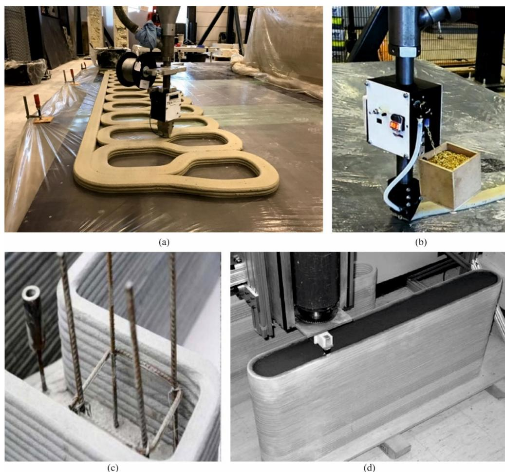
**Figure 6.** Different reinforcement methods for 3D-printed concrete (a) AM via introducing a steel cable into the concrete layer [63], (b) early version of reinforcement entrainment device [64], (c) contour crafting combined with vertical steel reinforcement [65], and (d) reinforcement in contour crafting [66].
