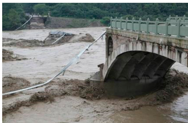
Figure 1. Collapsed Sichuan Panjiang Bridge [2].
