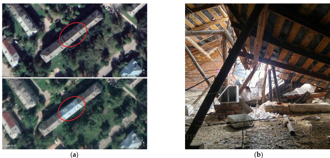
Figure 1. Partial roof collapse of a residential apartment building (15/2 Rihard Sorge Str., Tula) on 23 March 2018: (a) Google snapshot before the collapse on 15 September 2017 ( top ); snapshot after the collapse and a partial repair of the damaged roof on 24 August 2019 ( bottom ). The snapshot dated 12 October 2018 has worse quality. The affected part is outlined. (b) General view of the destruction. Photo from the site of IA Tula News ( https://newstula.ru/fn_349771.html (accessed on: 24 August 2021)).
