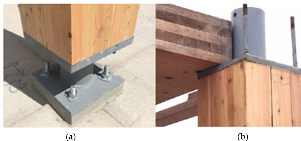
Figure 21. Column base connection (a) and floor support (b).
