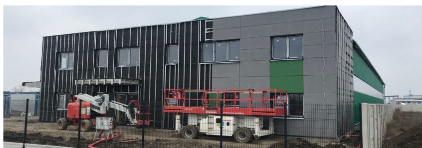
Figure 11. Real administrative building with ventilated facade.
