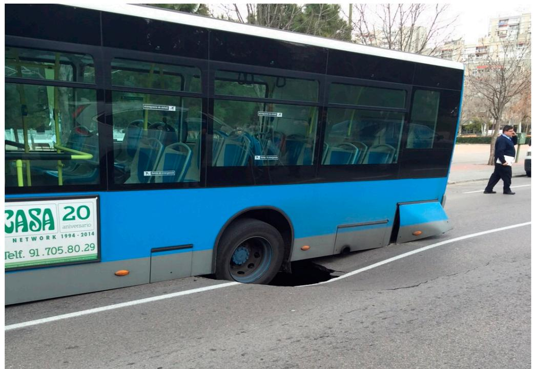
**Figure 2.** Sinking of a vial constructed of man-made due to sewer collapse.
