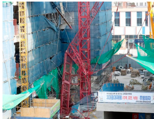
Figure 1. A 30 m T/C (tower crane) collapse at a construction site in Incheon, Korea [5].
