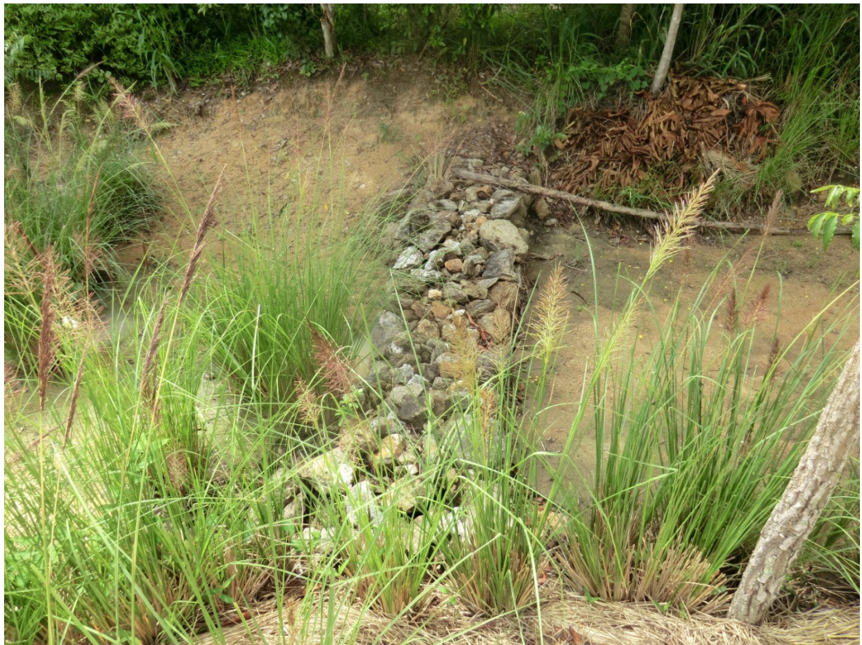
Figure 3. Erosion control measures including rock check dams and plantings of vetiver grass. Photo by Jonathan Long.
