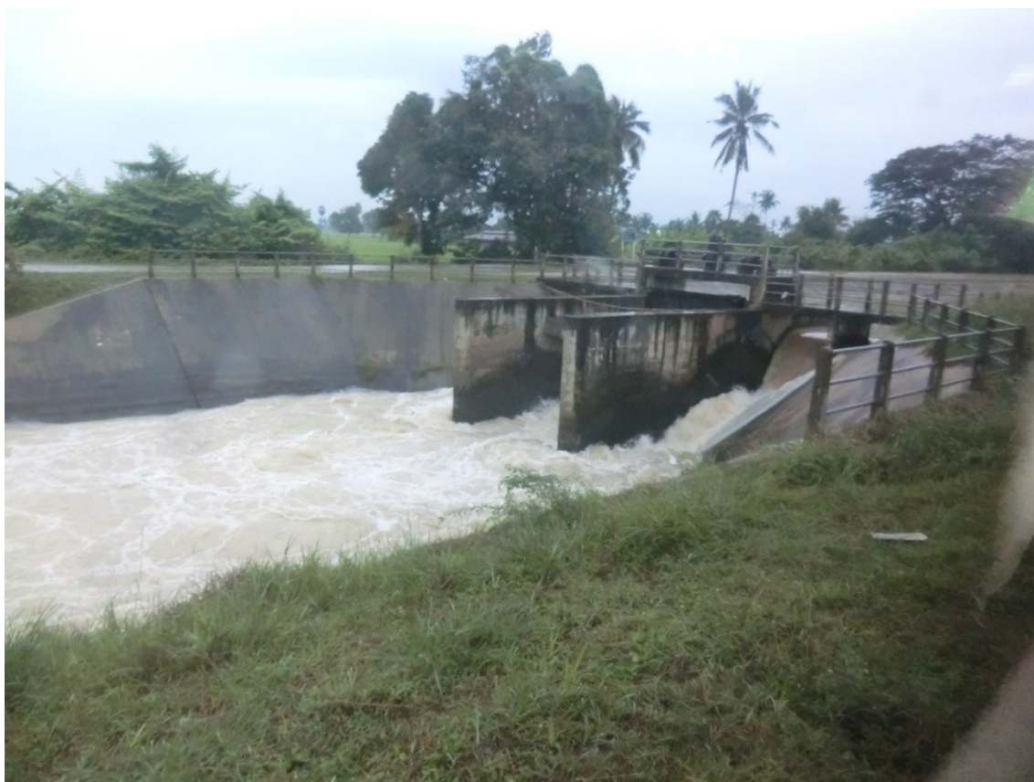
Figure 2. Water conveyance structure delivering water from storage reservoirs outside the SIEP watershed to downstream agriculture, cities, and tourism-related development. Photo by Jonathan Long.
