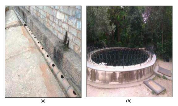
**Figure 9.** *Peisistratian* aqueduct: (**a**) branch of clay modular pipes near the Syntagma metro station in Athens (lids are missing); (**b**) contemporary mid-19th century terminal open pond in the National Garden, fed by continuous water flow from the *Peisistratian* aqueduct (photos by G. Antoniou).
