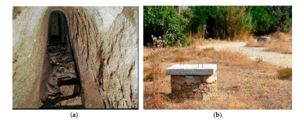
**Figure 12.** Roman underground aqueduct in the Aegean island of Rhodes, Greece: (**a**) part of the underground tunnel; (**b**) aligned shafts at the ground surface (photos by A. N. Angelakis).
