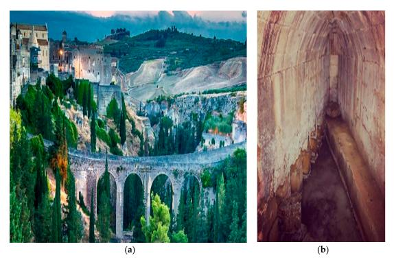
**Figure 23.** (a) The bridge carrying water to the town of Gravina in Puglia (on the left side of the gorge), after a 3.5 km-long course of the underground aqueduct "Madonna della stella"; (b) view of a segment of the underground aqueduct [72].
