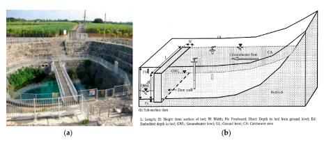
**Figure 27.** Underground dams: (**a**) Fukuzato underground dam [85]; (**b**) general sketch of an underground dam [84].
