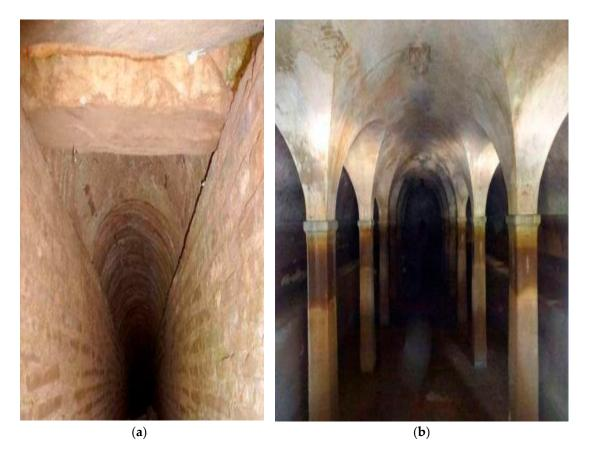
**Figure 14.** Parts of the Hadrian aqueduct: (**a**) underground tunnel near *Acharnes*, 10 km north of Athens at the foot of the *Parnitha* mountain; (**b**) terminal cistern, rebuilt during the 1870s (Photos by G. Antoniou).
