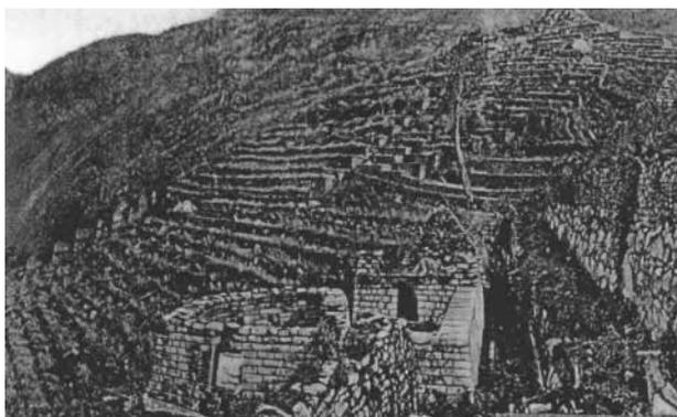
**Figure 6.** Machu Picchu Agricultural Terraces (by Hiram Bingham in 1912) showing tons of undamaged walls made by stone which resisted Landslides and earthquakes. Drainage systems (surface and subsurface) were built to manage average annual rainfall of 1940 mm [69].
