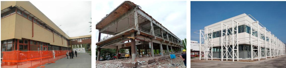
**Figure 4.** Steps of the seismic retrofit of the Magneti Marelli headquarters in Crevalcore, Italy.
