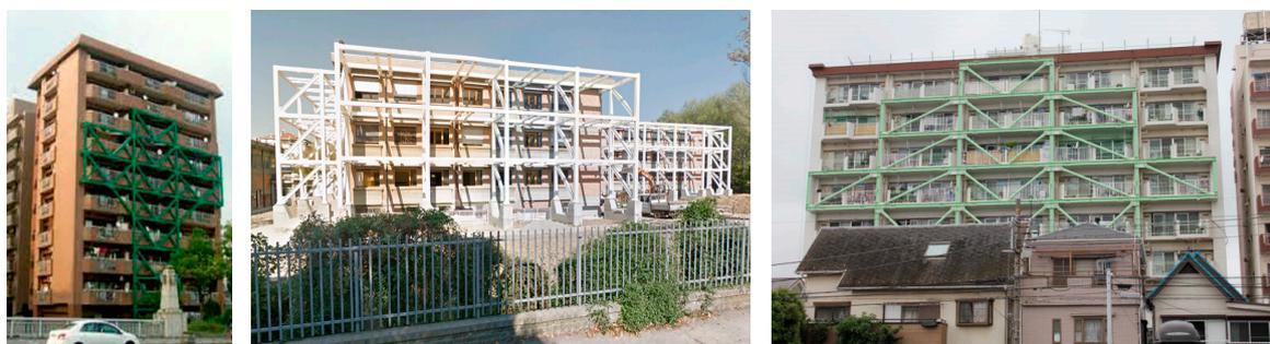
Figure 3. Examples of seismic retrofitting with steel exoskeletons.
