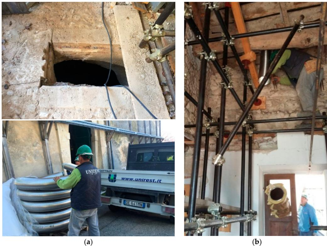
**Figure 9.** Preliminary steps for duct installation: (a) removal of the grid from the cellar window for the passage of the duct and storage in the site yard of the duct; (b) duct installation phase.
