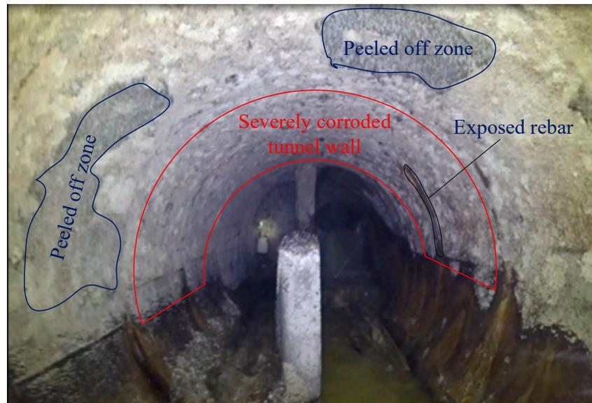
Figure 1. Corrosion conditions in a chamber located under 127 Street and 153 Avenue in Edmonton.
