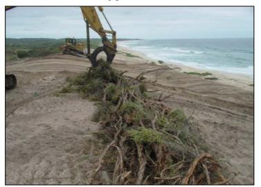
Figure 7. Coastal tea-tree being placed on the reconstructed dune crest.
