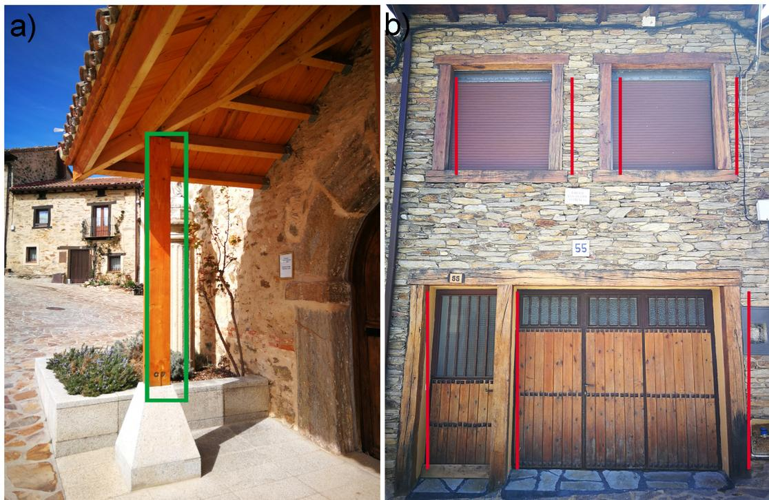
**Figure 1.** (a) Porch column of a church (Madrid) (green rectangle) and (b) pillar supports of a façade of a rural house (Madrid) (red lines).
