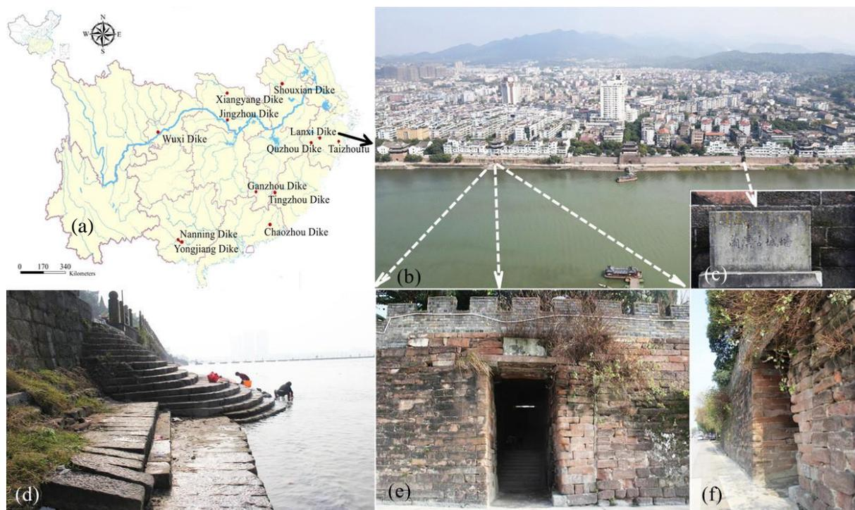
**Figure 1.** Characteristics of flood-controlled ancient dikes in South China. (a) Typical ancient dike distribution; (b) aerial view of Lanxi Ancient Dike; (c) ancient dike boundary stele; (d) ancient wharf; (e) city gate hole in ancient dike; (f) side view of ancient dike.
