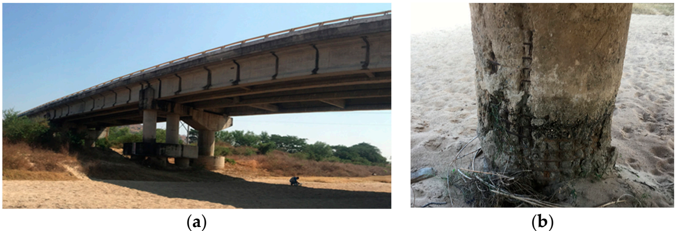
Figure 1. Bridge structure located near to Mexican Pacific coast: (a) longitudinal view and (b) structural element with deterioration.
