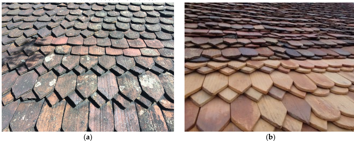
Figure 14. Different types of roof tiles: (a) historical; (b) new roof tiles in historic dimensions.
