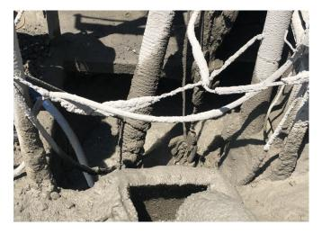
Figure 2. Concrete slurry water extraction.
