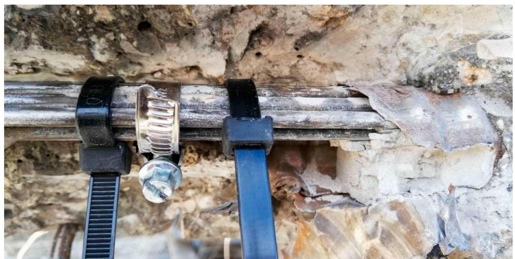
**Figure 4.** Prestressing wires after exposure (no signs of corrosion).
