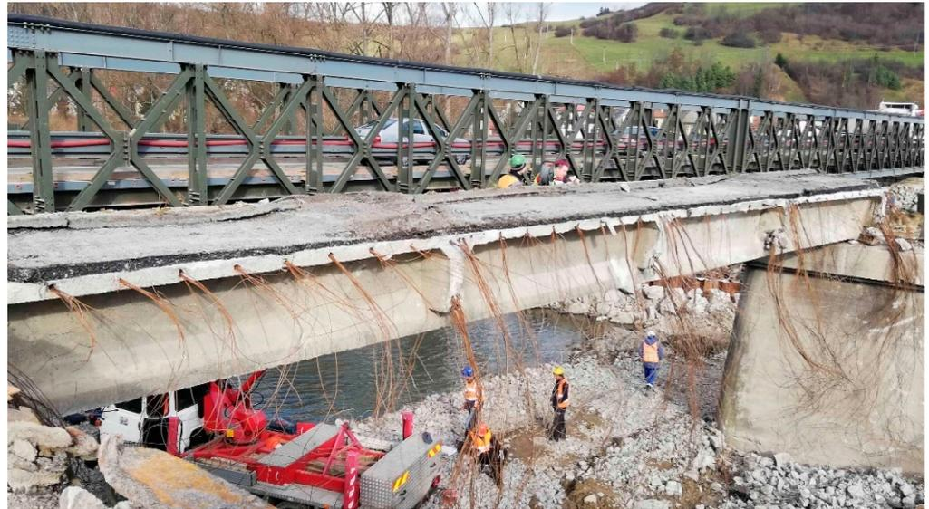
**Figure 3.** Material on the upper flange of the investigated post-tensioned concrete beam.
