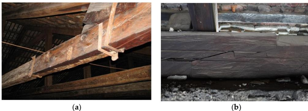
**Figure 4.** Examples of scarf and splice joining of wooden beams in existing buildings: (a) building in Italy, (b) building in Poland—13th century Czocho Castle in Sucha.
