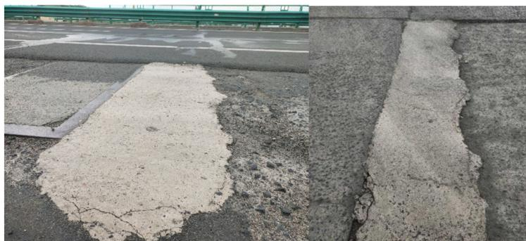
**Figure 19.** After nine months of service of the repaired pavement.
