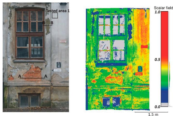
**Figure 1.** Part of the tobacco factory building—real photo on the left, point cloud on the right.
